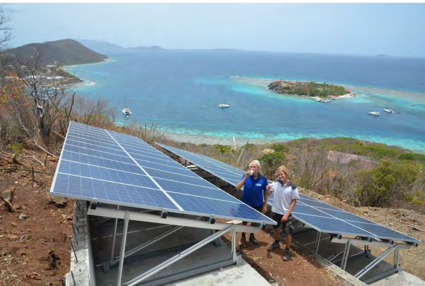
Figure 1 Founders at the solar panels of the installation on the Virgin Islands
